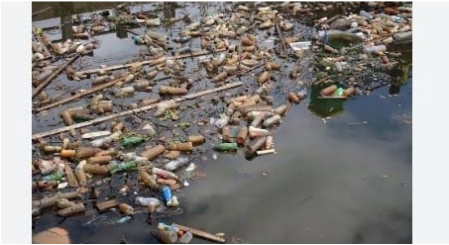
A polluted wastewater treatment facility near the Tshwane border, photographed on 9 July 2025. (Photo: L. Mokoena)
