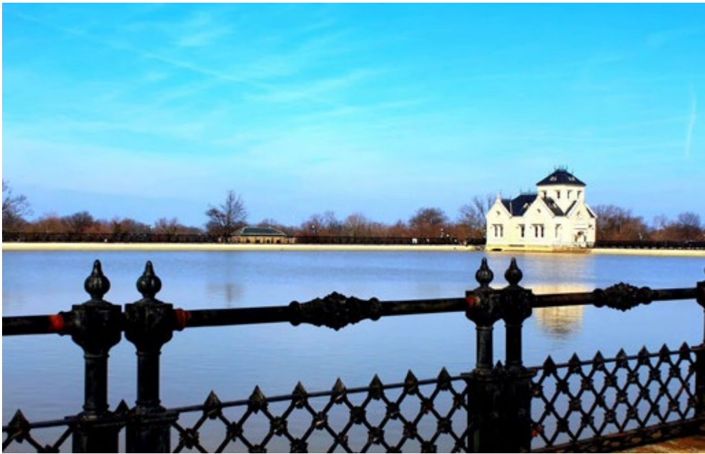
Figure 4: The Crescent Hill Water Filtration Plant, on a sunny day. Photo from “Louisville Family Fun”
