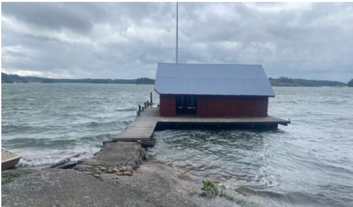
Boathouse during the storm, Nauvo. Photo: Alvin Ekelund, October 2025.
