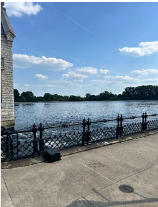
Figure 5: First reservoir of water held at Crescent Water Filtration Plant, full of water actively being filtered. September 19, 2025, Photo by Samuel Dobelstein.
